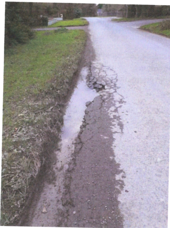
Figure 3.1 Photograph near The Meadows – typical failure of road due to existing traffic where the road is too narrow to accommodate large vehicles.
